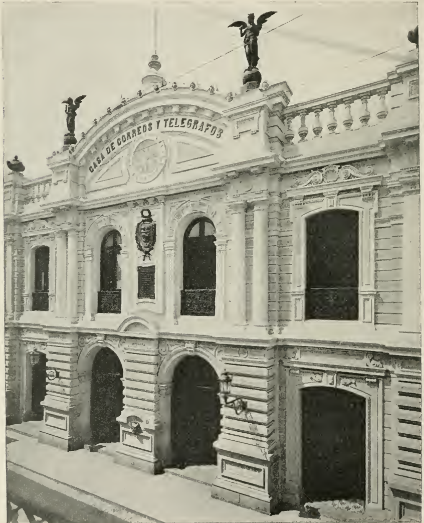
POST-OFFICE AND TELEGRAPH BUILDING, LIMA, PERU.
